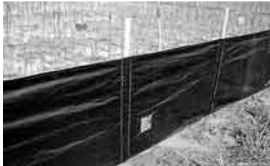
Figure 3.6 Plastic fence supported by bamboo posts.
